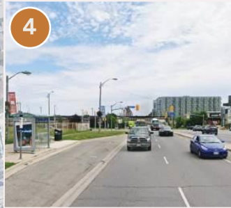
Existing condition along Wilson Avenue
